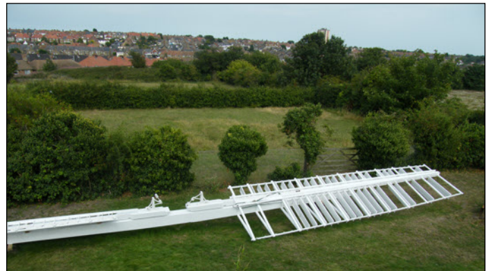
The refurbished second pair of sweeps awaiting re-fitting
