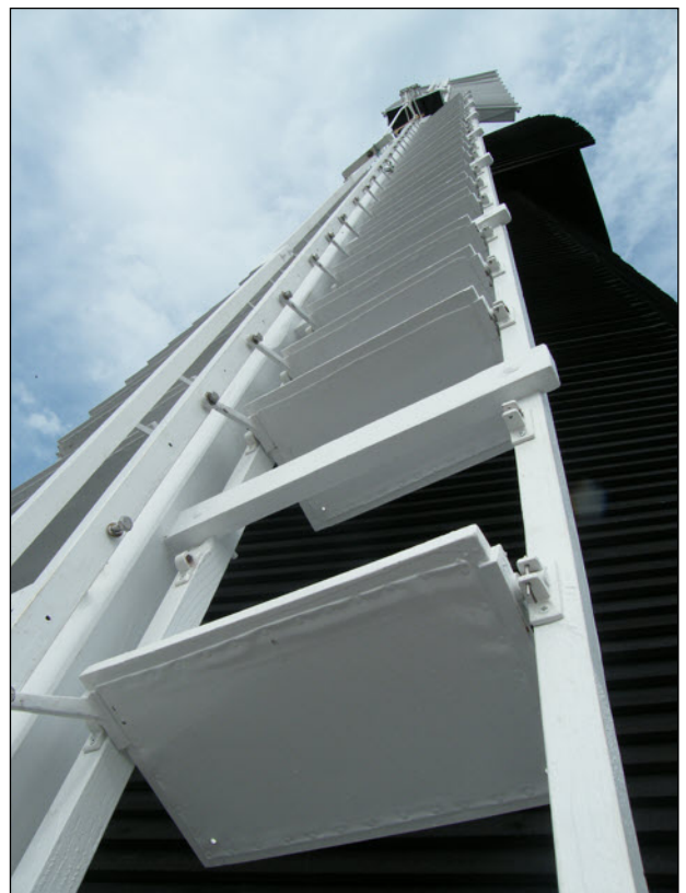
Some of the shutters on the pair of sweeps in situ on the day when these photographs were taken
